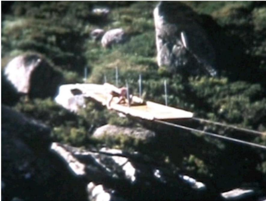
Photo No. 30 Securing wooden decking to supporting cables (John Turner 1957)
